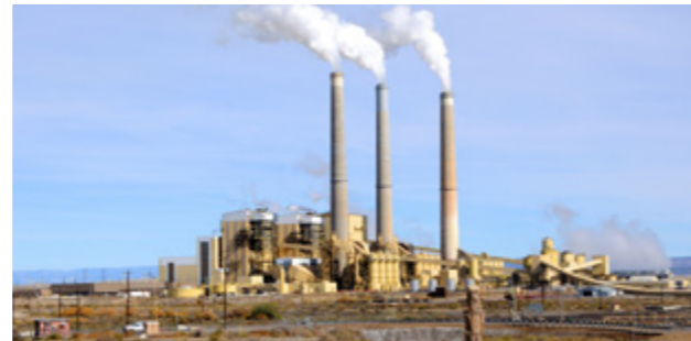
Jaguar Energy Power Plant Guatemala
